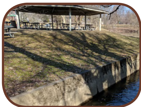
Concrete wall channelizing creek
