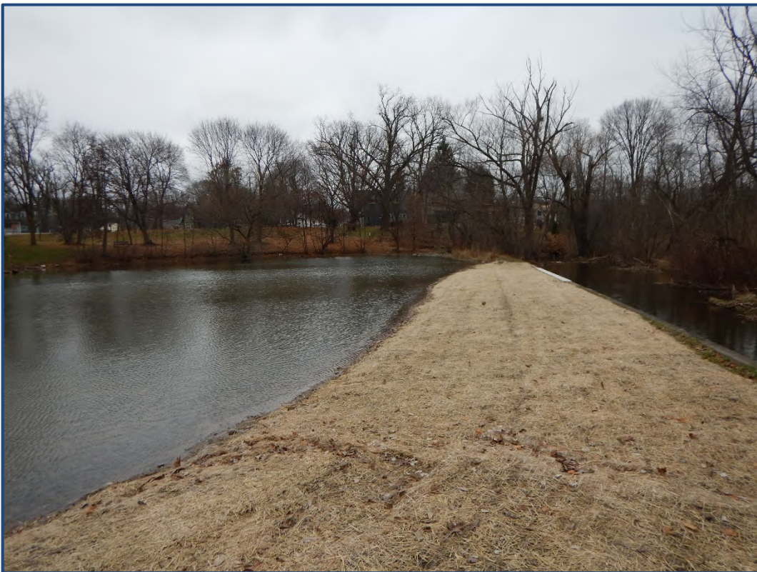
Photograph 4. Constructed pond with erosion control
